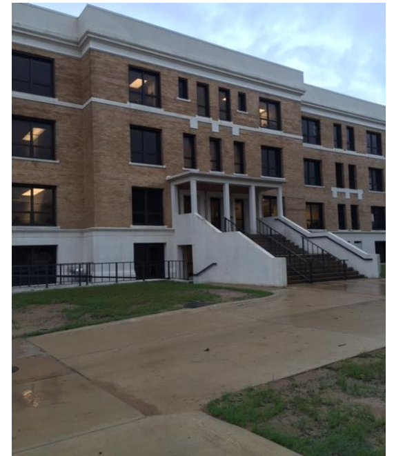
Milner Hall – North Entrance from Northside Parking Garage
