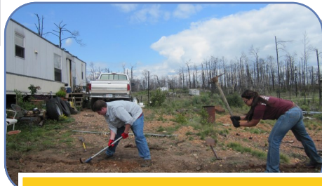
Fall '13 229 students dig trench for electrical conduit for fire survivors in Bastrop, still using an extension cord to get electricity to their home.
